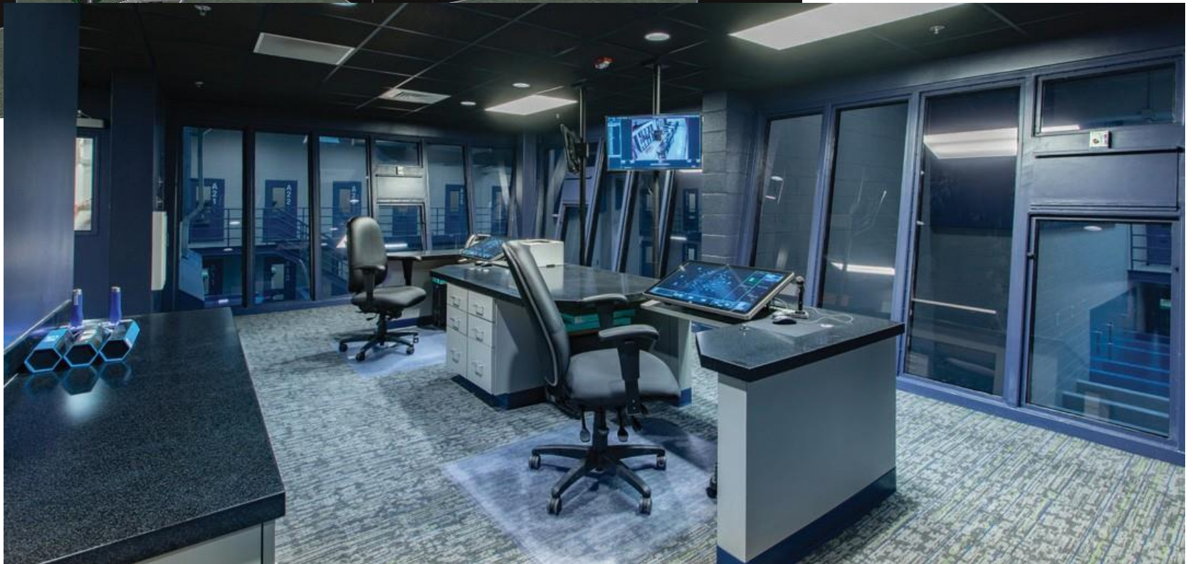
FINAL CONTROL ROOM DESIGN
